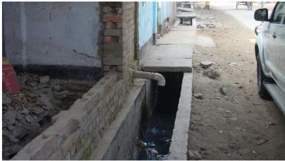
Rectangular urban drain with cover slabs
