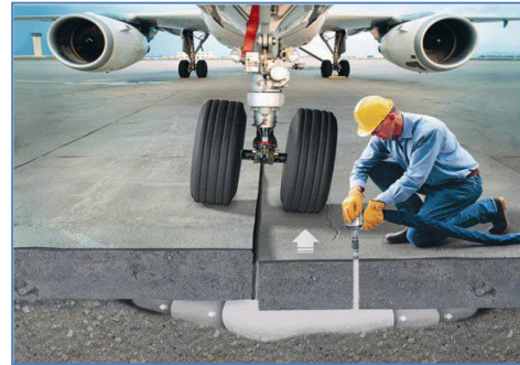
Slab stabilization
