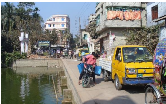
Urban retention pond
