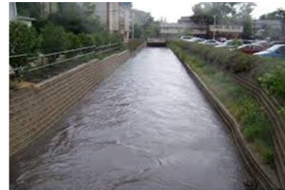
Well maintained urban drain
