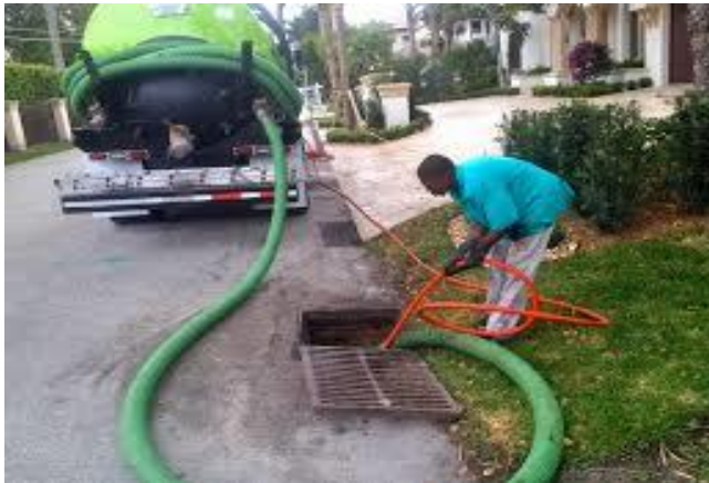
Cleaning a pipeline
