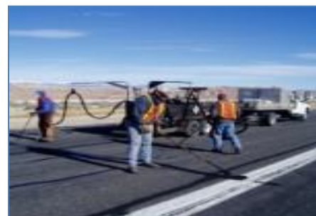
Crack filling
