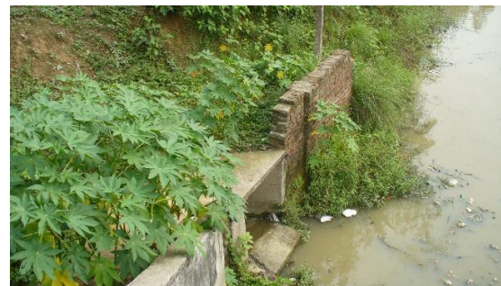
Outfall into a stream
