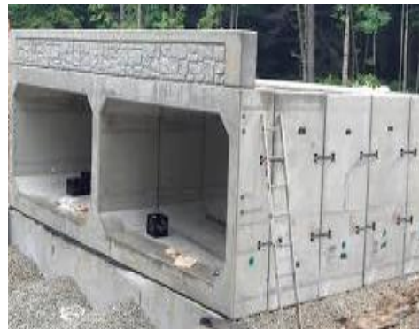
Twin concrete box culvert
