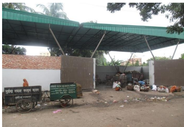
Secondary transfer station using traditional system of primary collection rickshaw van unloading and then loading to
