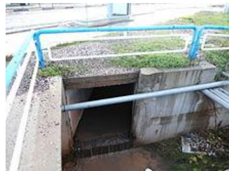
Drain under the main road empties into a bigger channel
