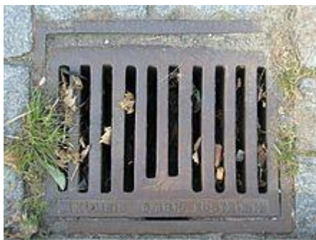
Cover Horizontal storm Inlet
