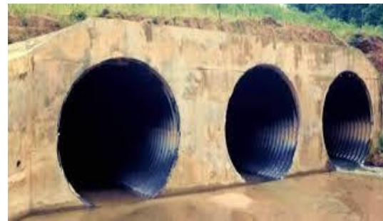
Corrugated iron culvert
