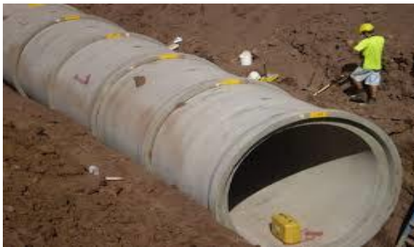
Concrete pipe culvert under construction
