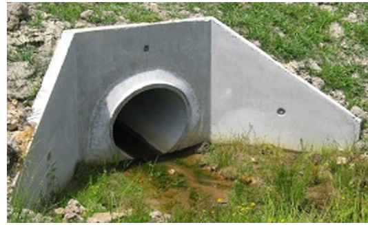
Reinforced concrete pipe culvert
