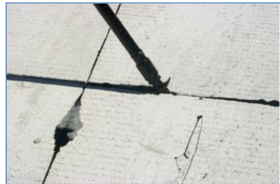
Joint sealing
