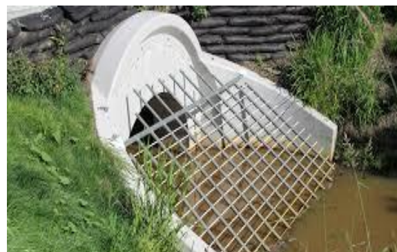
Grates help to keep a culvert clean
