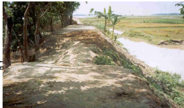
Figure-20 Settlement of Crest and side slope
