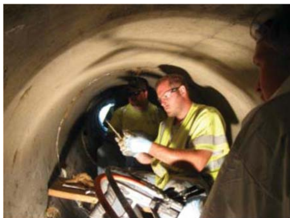
Sealing a pipe joint from the inside with activated oakum (jute fibers soaked with a resin)
