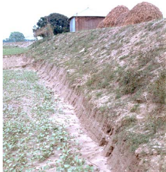
Figure-22 Cutting of Toe of Embankment
