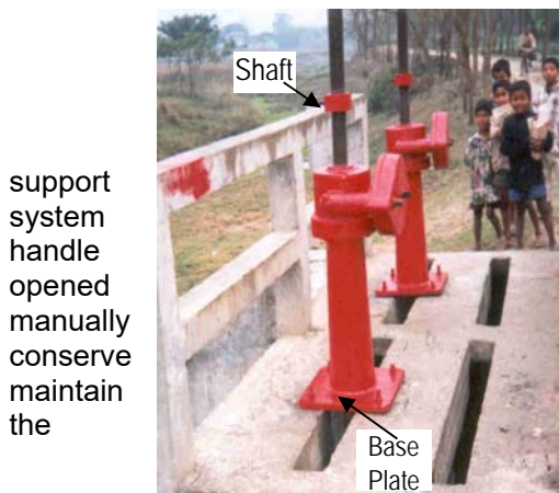
Figure-13 Raising of Vertical Gate
