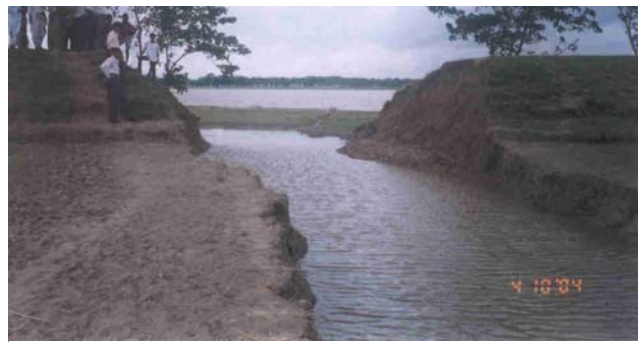
Figure-33 Embankment Breaching
